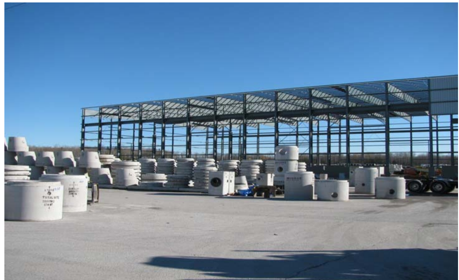
Munro Plant Expansion Under Construction in September 2010
