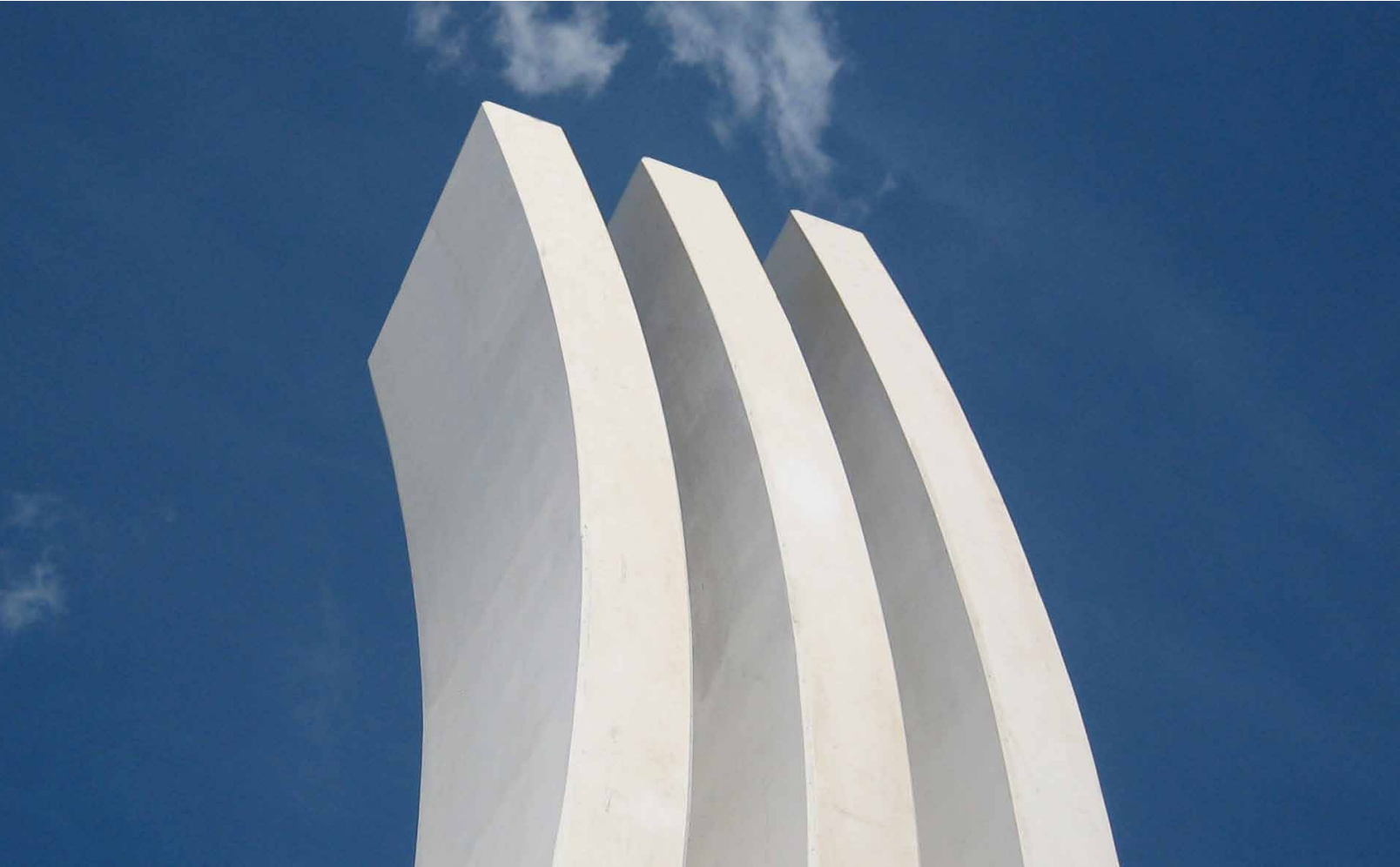
THE I-35 GATEWAY MONUMENTS, MINNESOTA. Built using photocatalytic concrete. Designed by Oslund and Associates.
